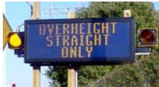
Overhead height warning system installed in Milwaukee, WI at the I-43 bridges over General Mitchell Boulevard.
