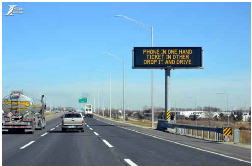
A new Dynamic Message Sign provides valuable traveler information along Illinois Route 390.
